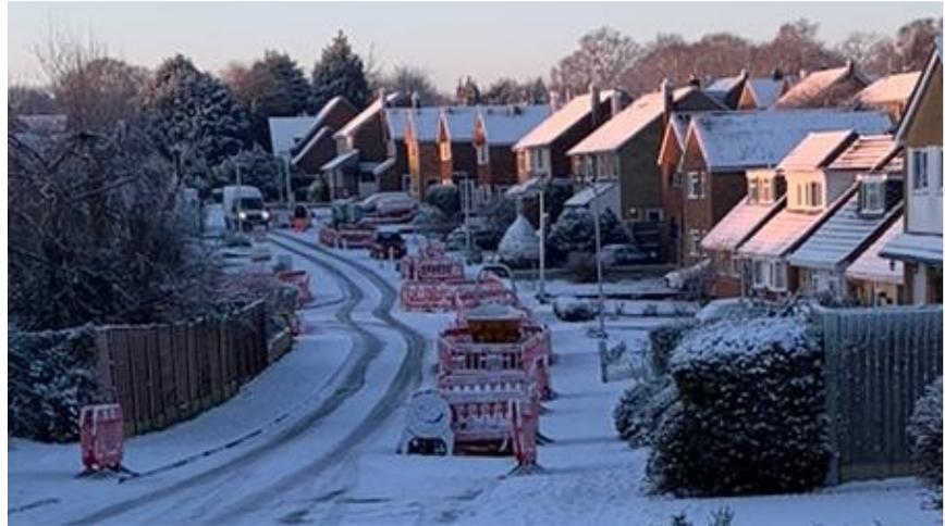
This scheme was carried out to rehabilitate existing water mains in the Draycote area of Rugby and involved the replacement of 10,224m of 75mm - 250mm dia Asbestos Cement, Cast Iron and UPC Water Mains in 23 separate roads under Severn Trent Water's AMP7 Lot 2 'Build Only' framework.
